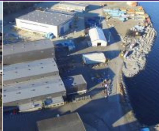
Bergen Quay Side facilities
