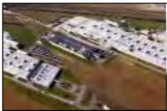
TMUK – Engine Plant
